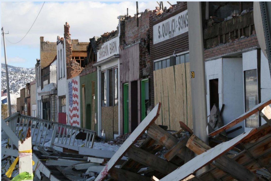
Image of 2008 Wells Earthquake Damage by Nevada Bureau of Mines and Geology, Presentation on Seismic Risk of Unreinforced Masonry Buildings in Nevada, October 2019
